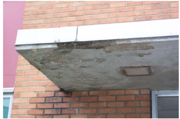
Southwest entry canopy
