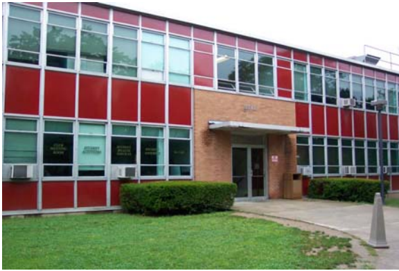
Exterior at south façade
