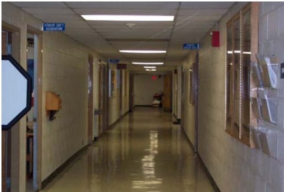
Ground floor corridor looking east
