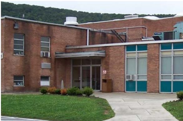
Lobby looking east
