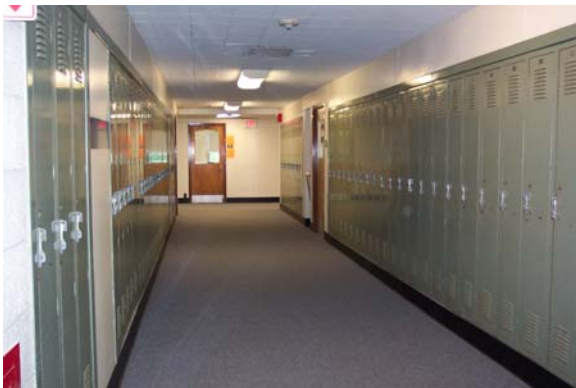
Second Floor Corridor, looking west
