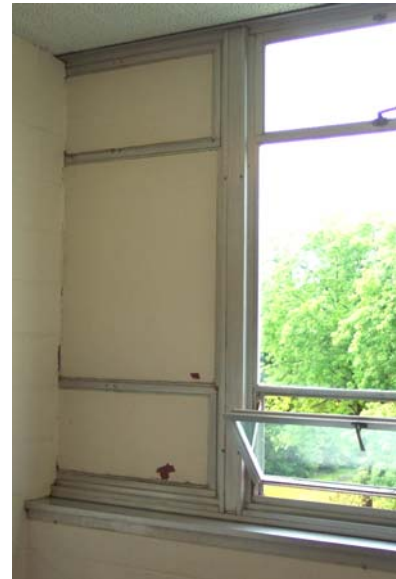
Window at Second Floor Stair Landing
