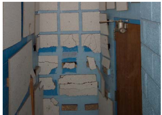
Vestibule at Theatre SC101
