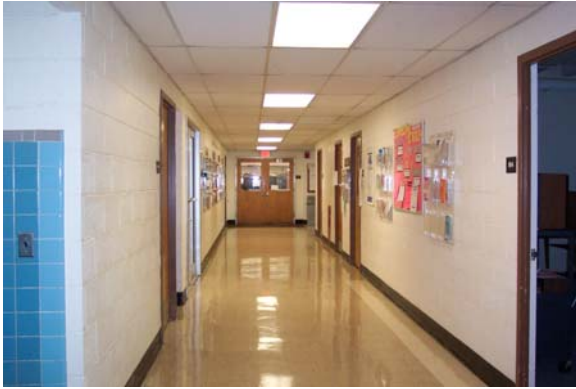
Ground Floor Corridor, looking east
